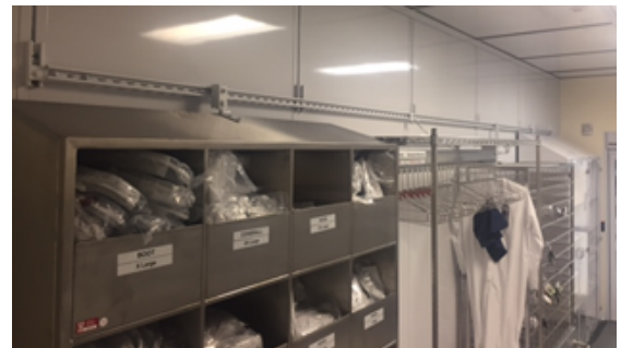
Newly installed shelving brackets prevent tipping
